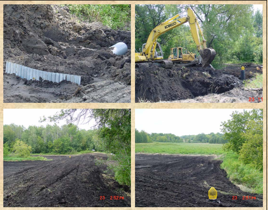
(Right) Clockwise from top left: (1) Seating of pipe with anti-seep diaphragm attached (2) back-filling around structure (3) view of intake and drained wetland (4) completed dam ready to be seeded. (Above) Same wetland 11 months later.
